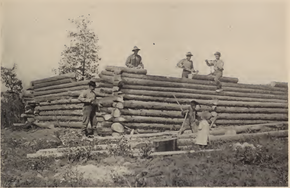
MR. McINTOSH AND BOYS AT WORK ON THE BUILDING
